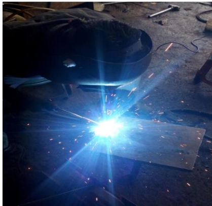
Welding Process is being done
